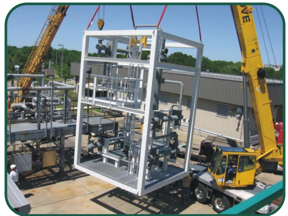
Installation of PTU
